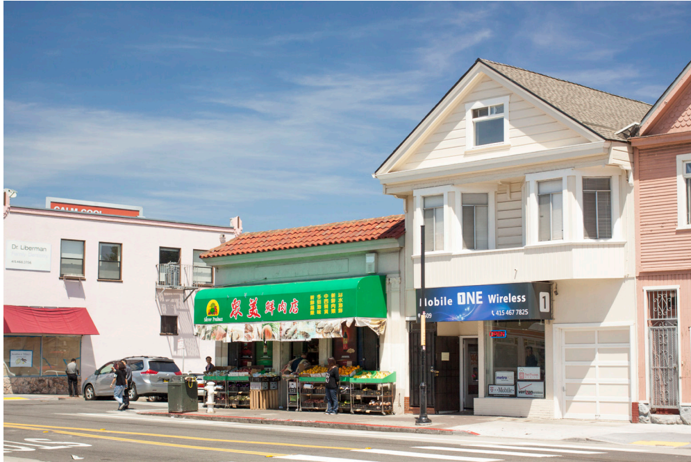
Figure 17: San Bruno and Thornton Stop, Existing. Author photo.
